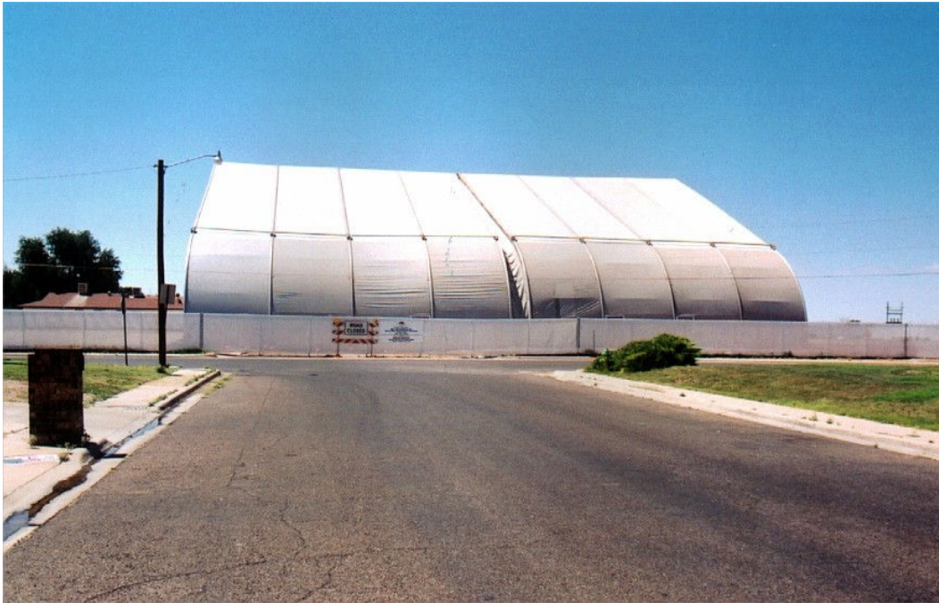
Figure 3. Close up Photograph of Tank Battery in Relation to one of the two exposed Streets.
